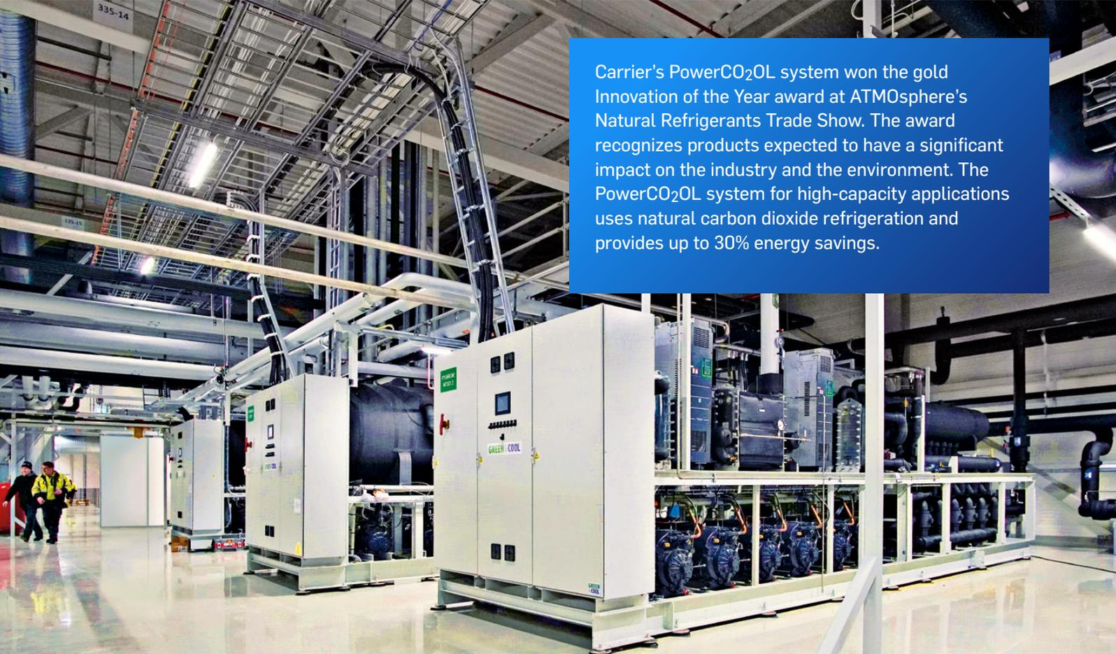
Carrier's PowerCO<sub>2</sub>OL system won the gold Innovation of the Year award at ATMosphere's Natural Refrigerants Trade Show. The award recognizes products expected to have a significant impact on the industry and the environment. The PowerCO<sub>2</sub>OL system for high-capacity applications uses natural carbon dioxide refrigeration and provides up to 30% energy savings.
